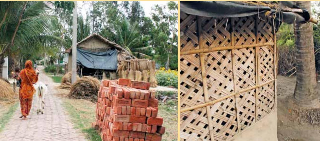
*From left to right: Harvesting and cleaning of straw, a highly sustainable resource, suitable for the self-build of artefacts, planned by the project; Typical local building technology; A wall made of bamboo, a fairly flexible material, available in large quantities, and used in traditional local construction*
